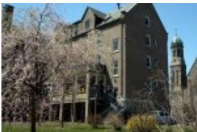
Back of the building
